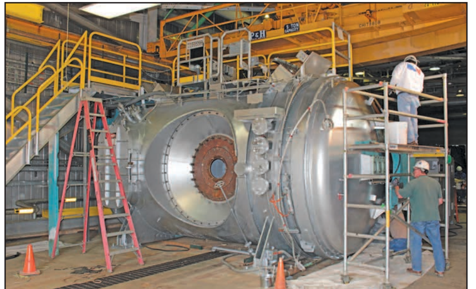
The AEDC arc heater undergoes significant upgrades in support of advanced hypersonic systems. This photo depicts upgrades conducted for the H2 test cell. In addition to the heater upgrade and other improvements, a new coat of paint was applied to the test cell. (AEDC photos)
